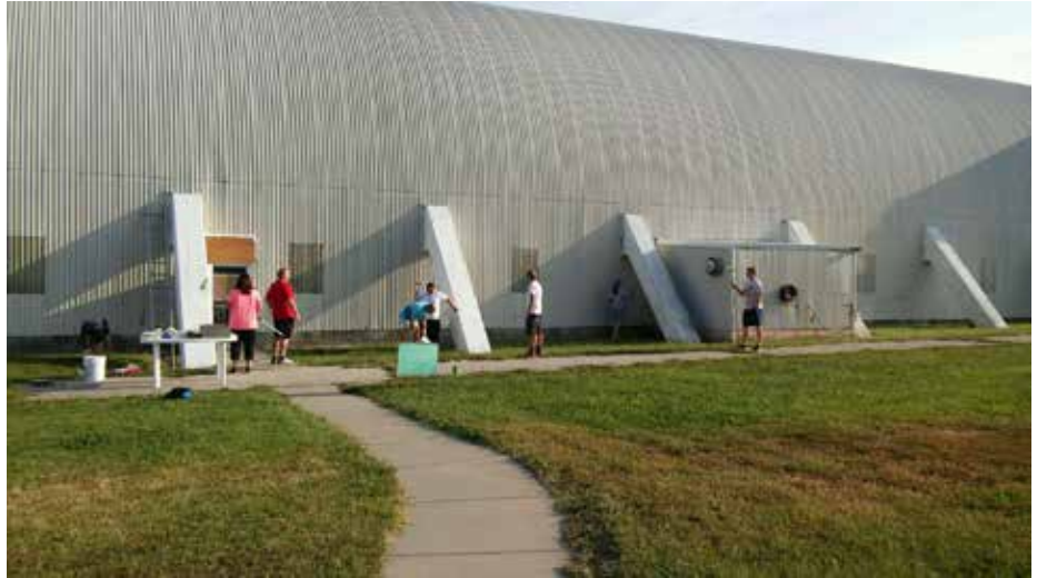
Auburn Troop 117 scouts paint buttresses on hangar 602 (photo by Kevin Drewelow)
